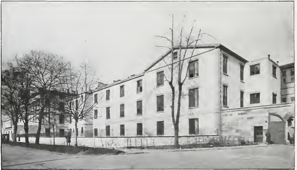
FIG. 182.—General Hospital No. 22, Philadelphia, Pa.
